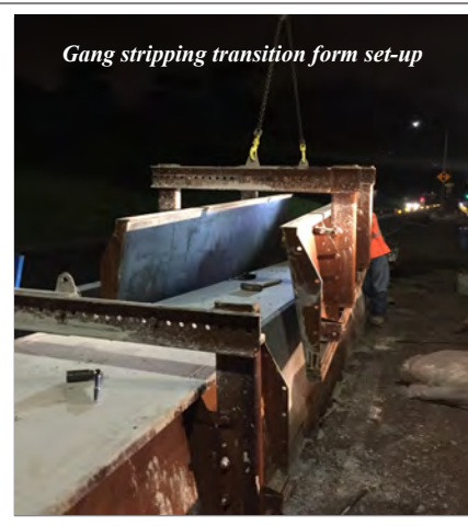
Transition forming from 9 1/4” top thickness to 54” wide to accommodate light posts
