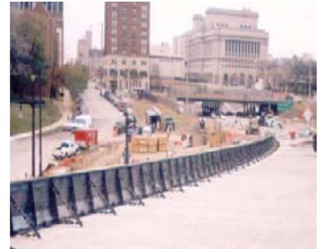
Barrier forms being used to form long merge lanes with gradual radius.
