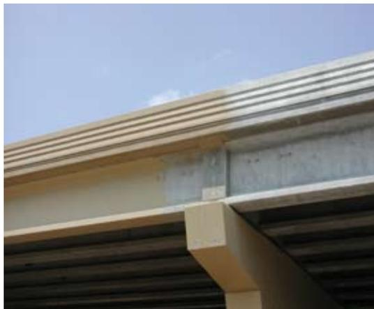
Metal Forms Corp. added a special façade feature to its standard concrete barrier to give an element of style on parapets throughout the Marquette Interchange being reconstructed in downtown Milwaukee. Finished surfaces are stained to enhance appearance. Contrast between finished and unfinished areas can be seen here.
