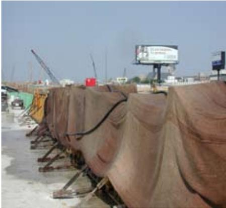
Parapets undergo a seven-day wet cure under burlap to develop optimum strength and durability
