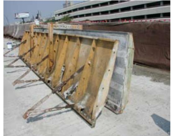
Façade form profile can be seen inside right side of parapet barrier form. Close up shows typical form aligner assembly that provides both vertical and horizontal form alignment. Also shown are moment arms, which allow Marquette Constructors to keep the forms together when stripping and recycle them for faster pours.
