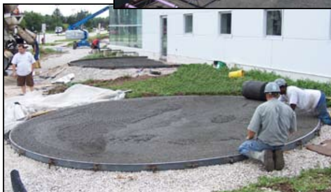
Forming car pads with pervious concrete
