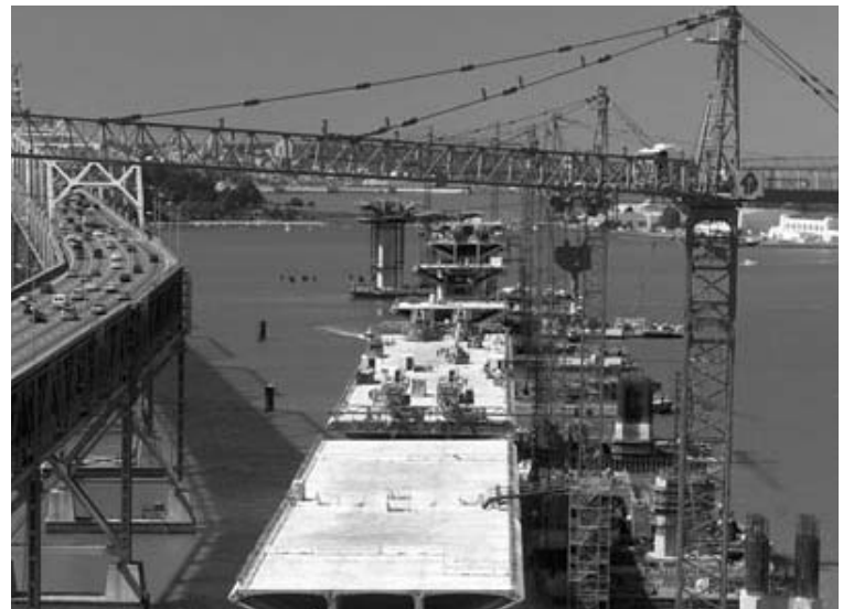
Metal Forms built a customized Speed Screed® for the Bay Bridge.
