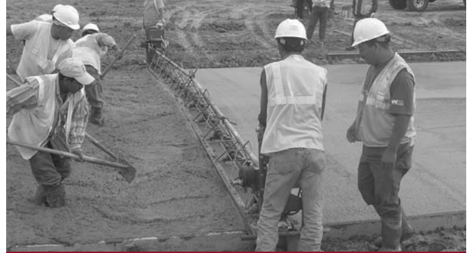
An MFC screed paves a new road in Texas.
