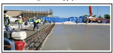
Mike Burton, of Reinforcing Steel Supply (RSS), snapped these photos of Hellas Construction using a Speed Screed® Heavy-Duty model on an athletic facility for the Georgetown Ind. School District.. (TX)
